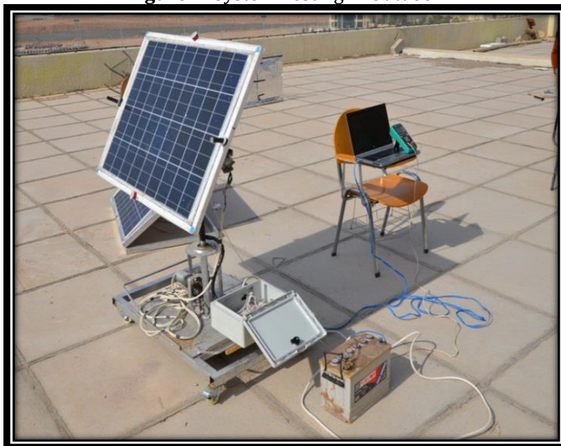
Figure 4: System Testing in Outdoor.
